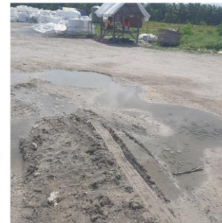
Photo 1: Storm water trapped.
