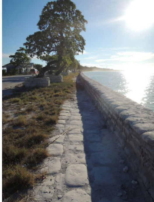
Figure 1 KAP-II sea wall in South Tarawa including apron.
