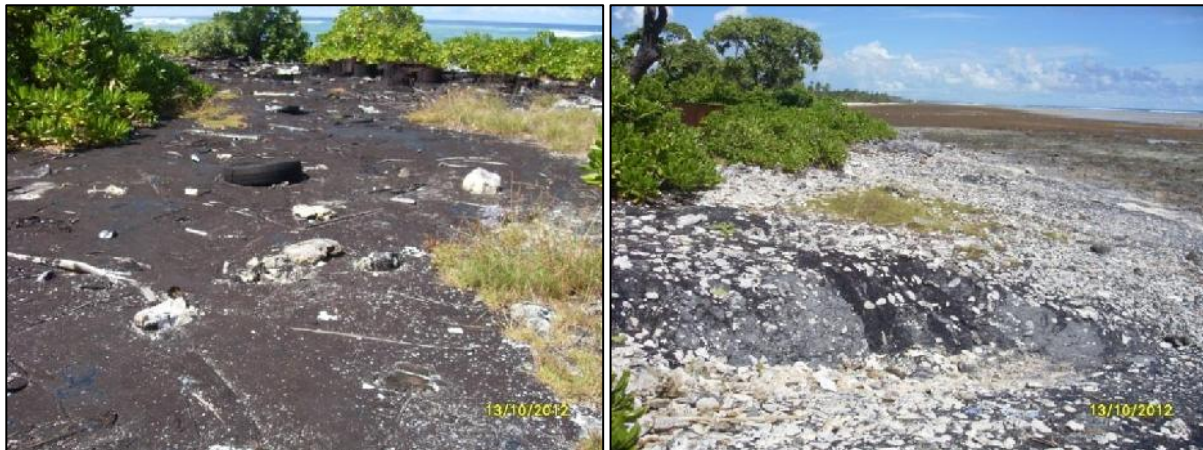
Figure 13 Bitumen dump adjacent to runway (north eastern corner) showing extent and spill onto beach
